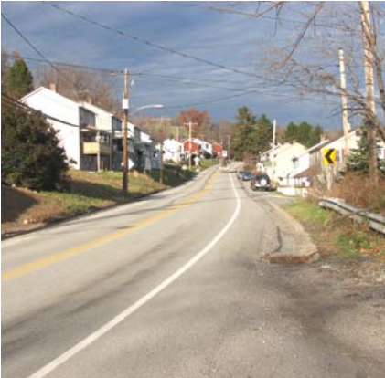
Figure 3.5: Waterman, in Center Township, is an example of a Village Center.
