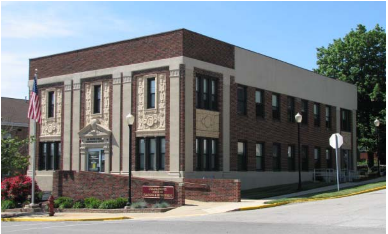
Figure: 5.15: The Indiana County Office of Planning and Development is in a historic building in Indiana Borough that has been renovated to provide two entrances that are accessible for all users. It also has bicycle parking available for visitors and employees.
