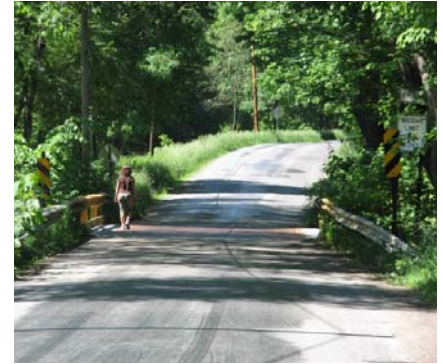
Figure 4.18: Martin Road sees a significant amount of pedestrian and bicycle traffic , but lacks formal infrastructure for safe travel.
