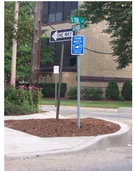
Figure 4.14: A completed Safe Routes to School project near Horace Mann Elementary School in Indiana Borough.
