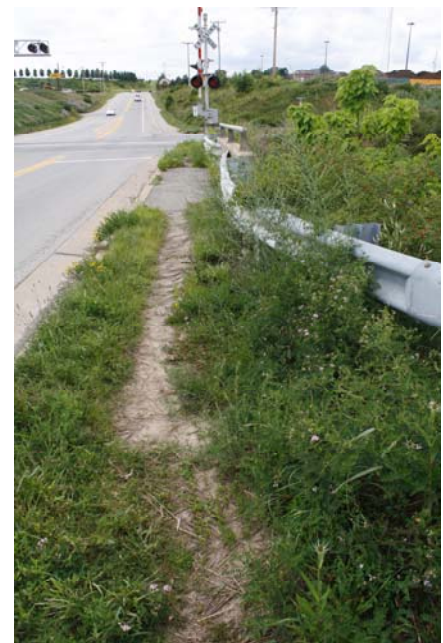
Figure 4.5: It is easy to see that there is a need for a sidewalk in this location.
