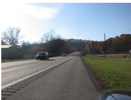
Figure 4.8: A wide shoulder such as this on roadways can provide a safe travel space for cyclists and pedestrians where it is not possible to provide a dedicated lane for them.
