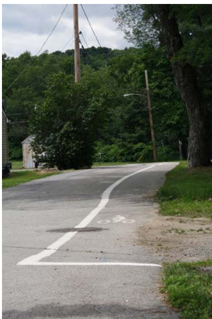
Figure 4.6: A bike lane that links two sections of the Hoodlebug Trail in Homer City Borough. This is one of only two bike lanes in the County. Together, they total less than 1 mile.
