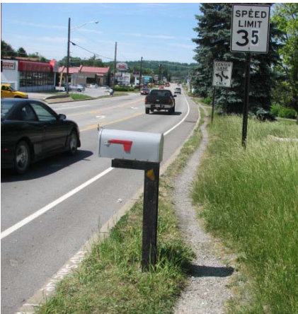
Figure 4.17: Oakland Ave. in White Township does not sufficiently support pedestrian mobility as evidenced by this “goat path.”
